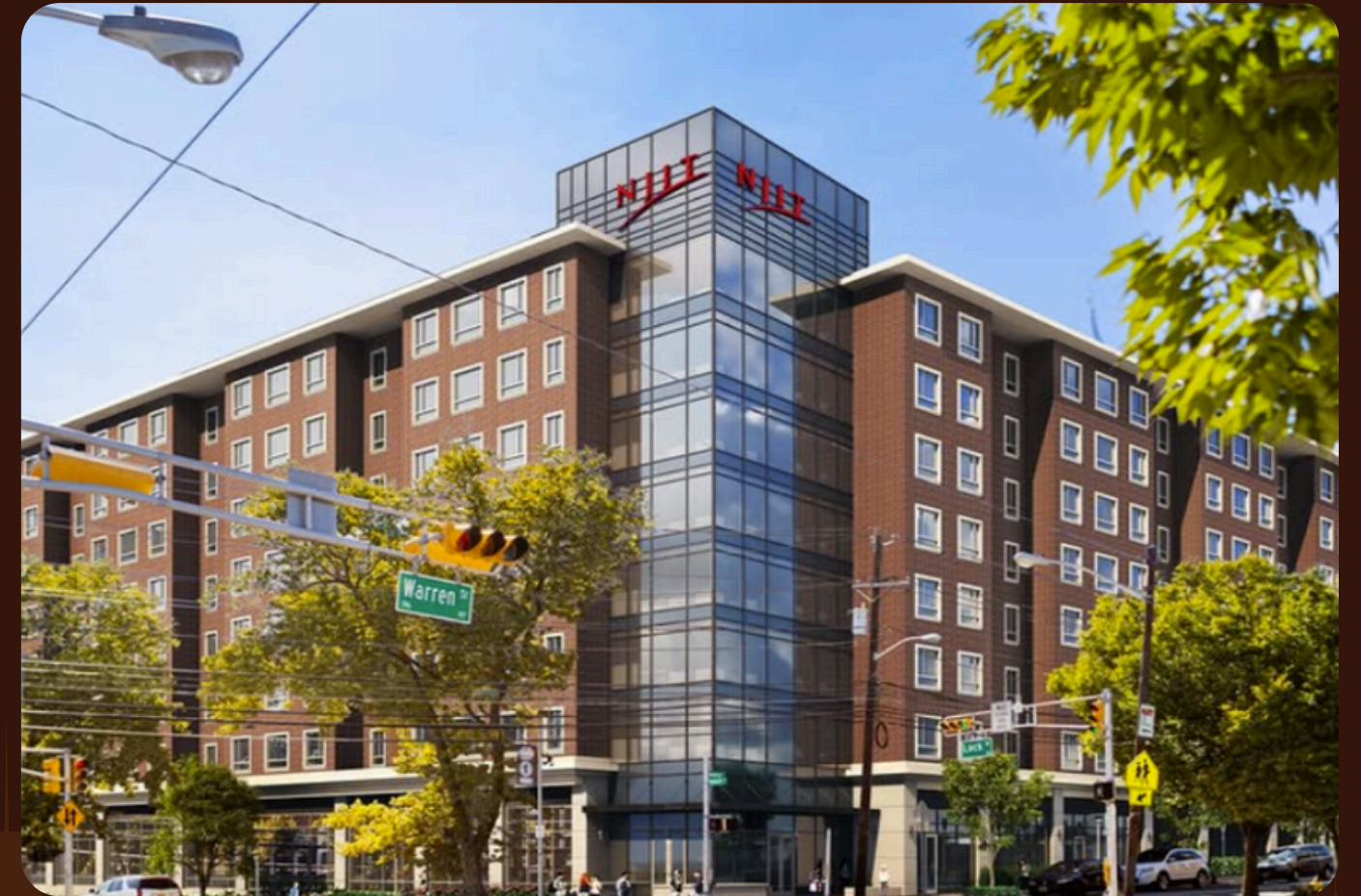
Maple Residence Halls
